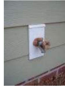
Outdoor faucets with built in backflow protection
