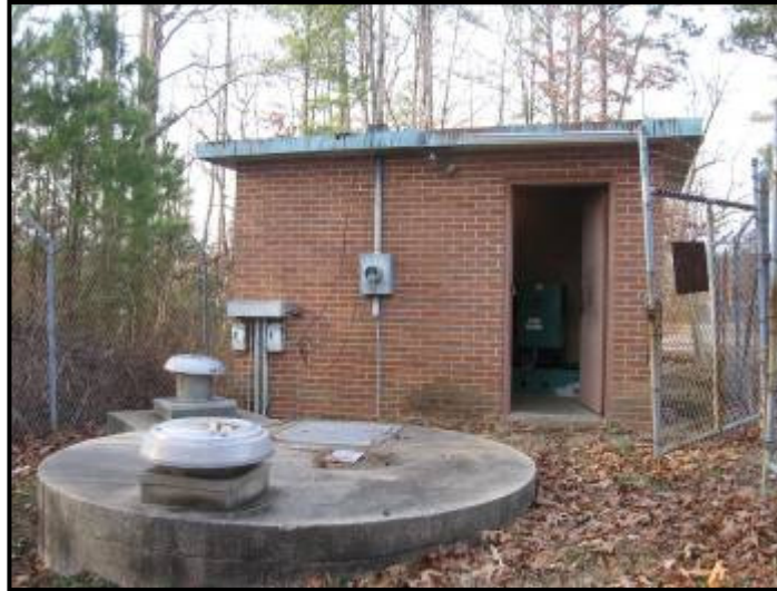
Figure 8 – School Street Sewage Pumping Station
