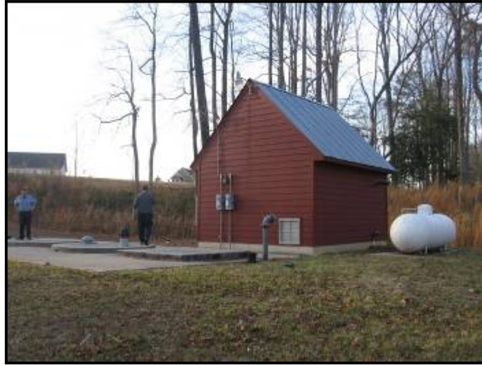
Figure 10 – Hills Quarter Sewage Pumping Station
