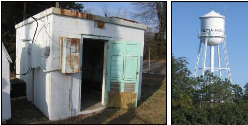
Figure 4 – Church Street Well Pump House Exterior and Elevated Tank
